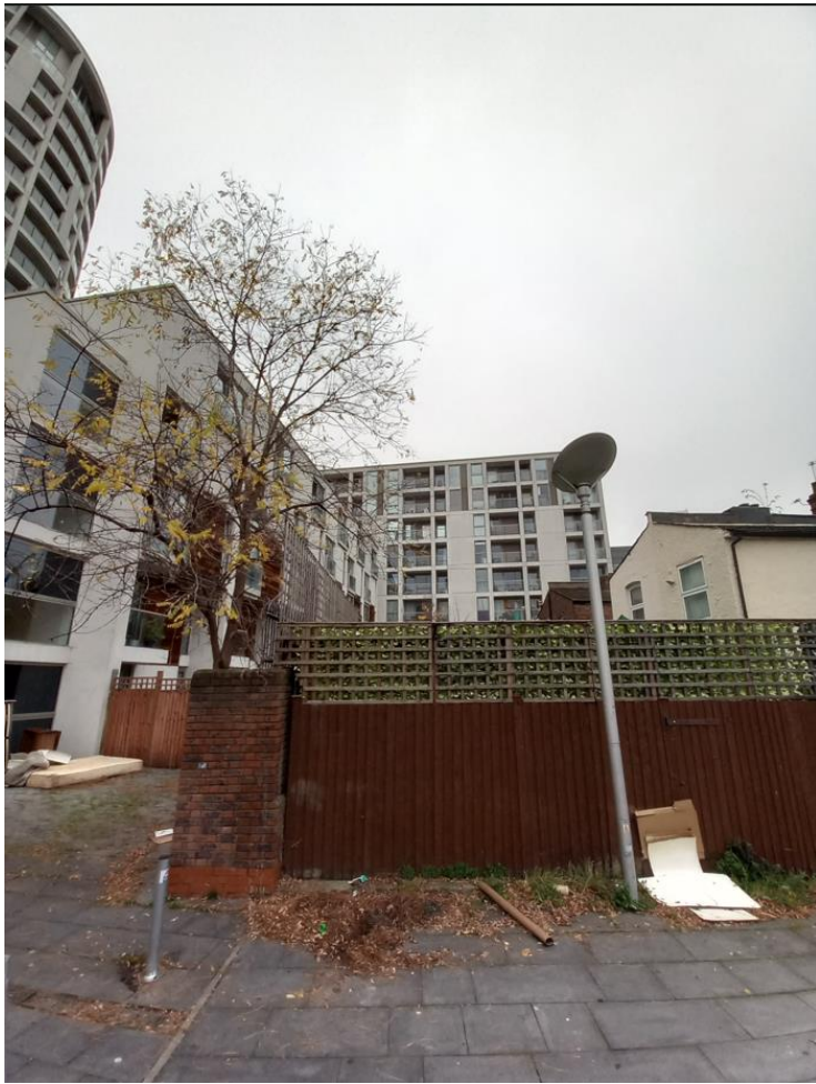
West Elevation. Photo taken on pedestrian walkway between Mellish Street and Boston House.
